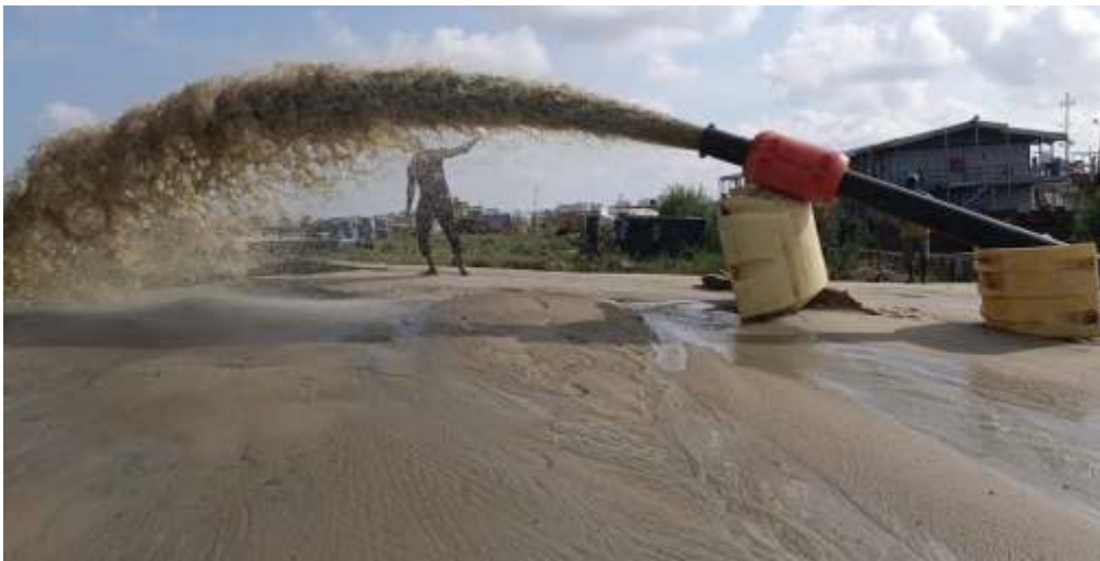
Fengsheng 01 high velocity projectile discharge at Lekki foreshore
