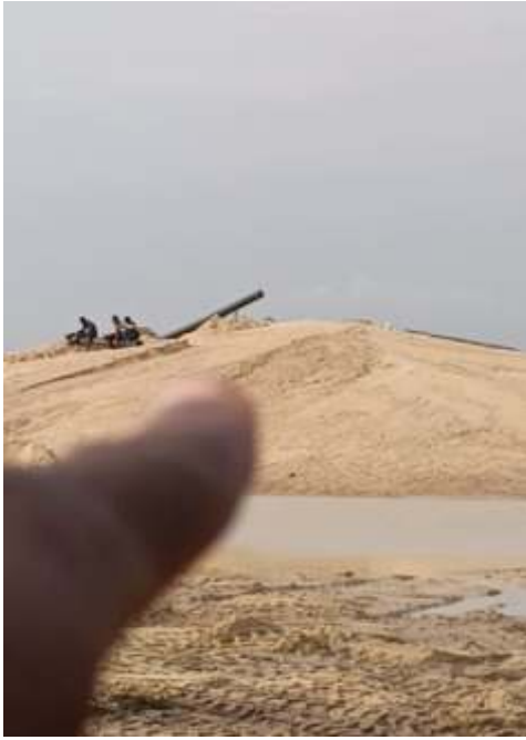
Stockpile pyramid after discharge
